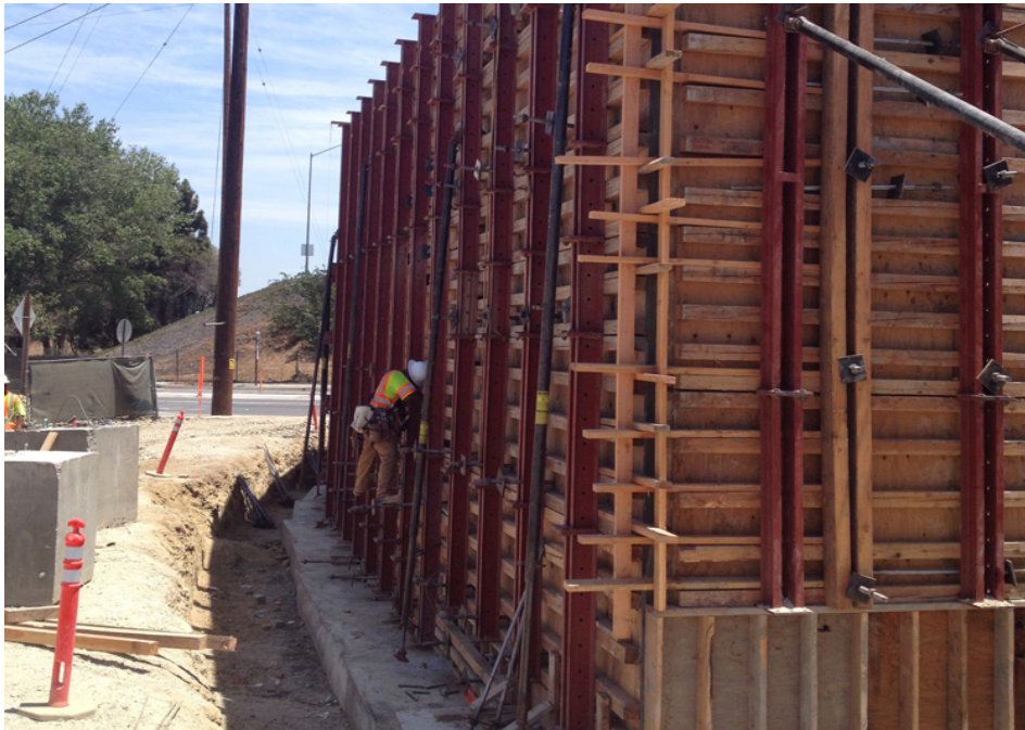
Crews conduct a lean concrete pour for the widening/realignment of Southbound I-405 On-Ramp at Wilmington Avenue.
